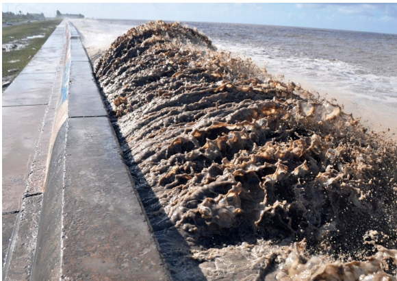
Waves breaking on unprotected section of seawall
