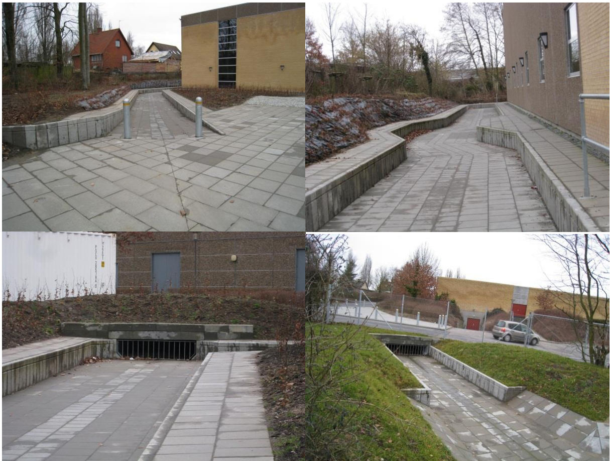
Figure A. 11 Photos from the area after terrain regulation
