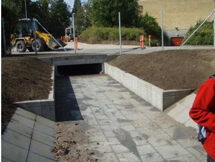
Figure 5.10 Relief channel to reduce flooding at Sports Park in Odense, established in 2008
